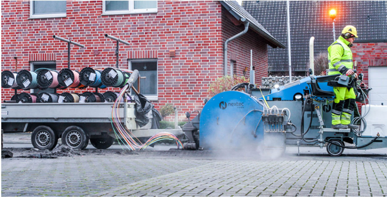
Figure: Microtrenching and backfilling of a microtrench post cable installation 19
