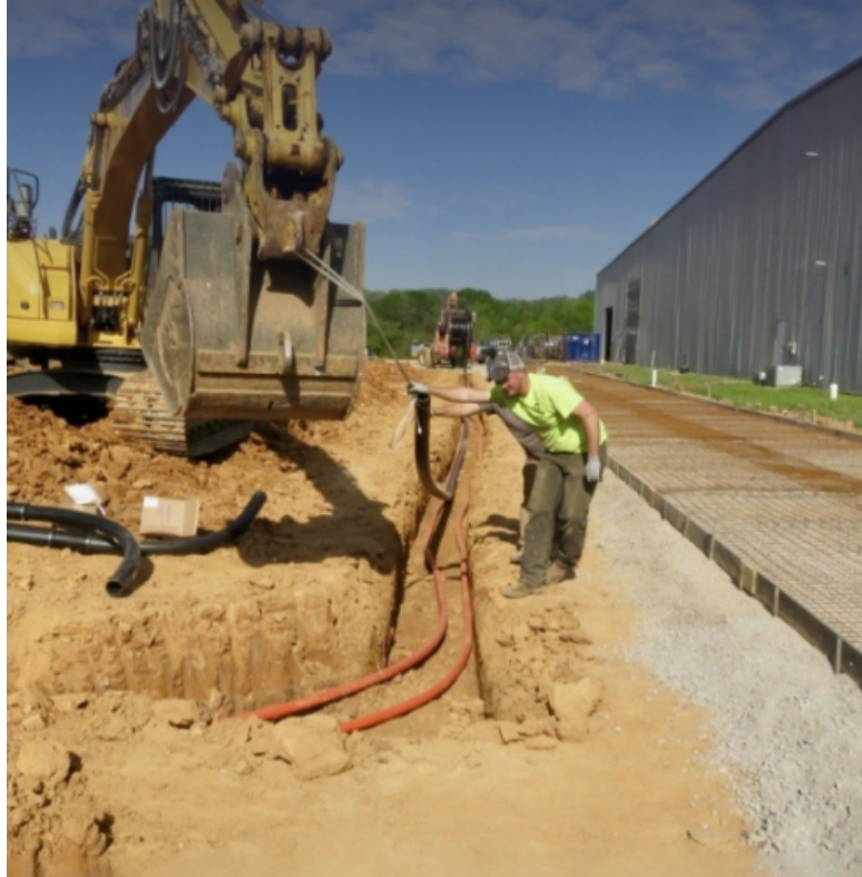
Figure: Fiber optic conduit laid in a joint trench 18
